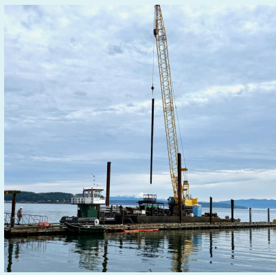
Crane removes old wood pilings
