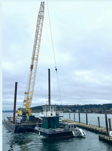
Dock repair barge arrives
